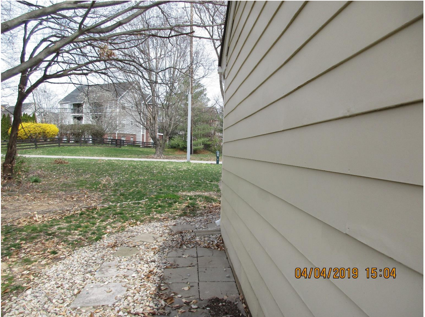
Variance area looking toward Old Springdale Road.
