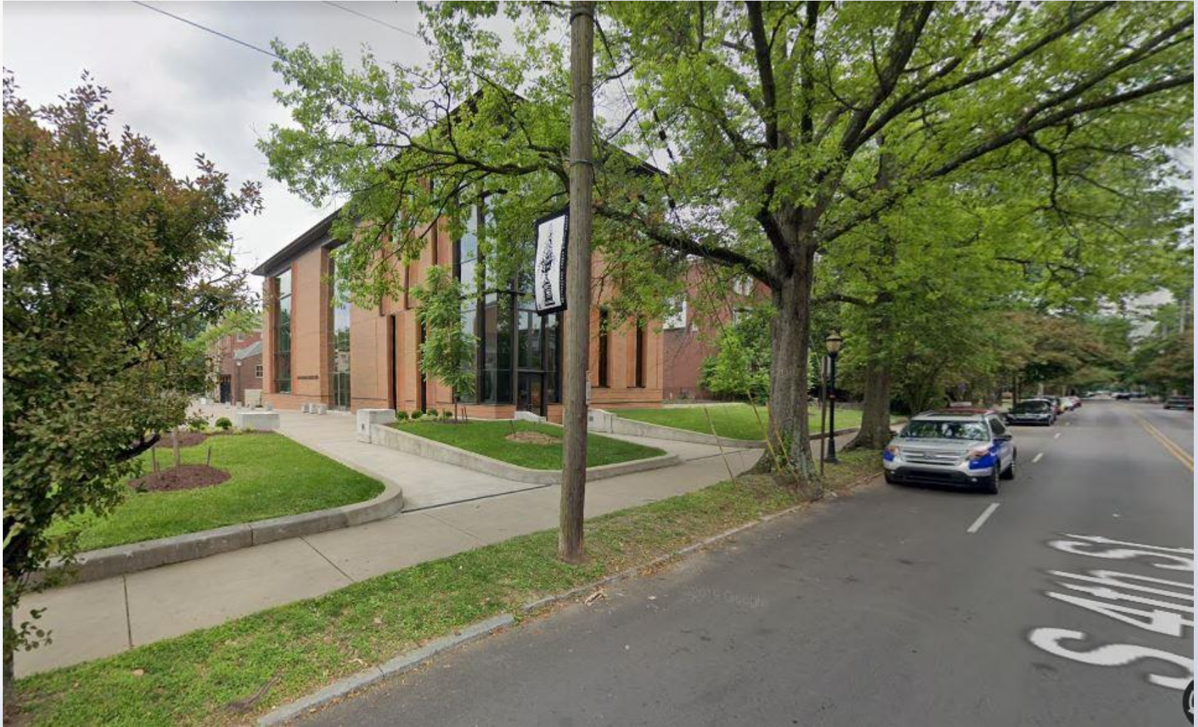
Site from S. 4th Street
