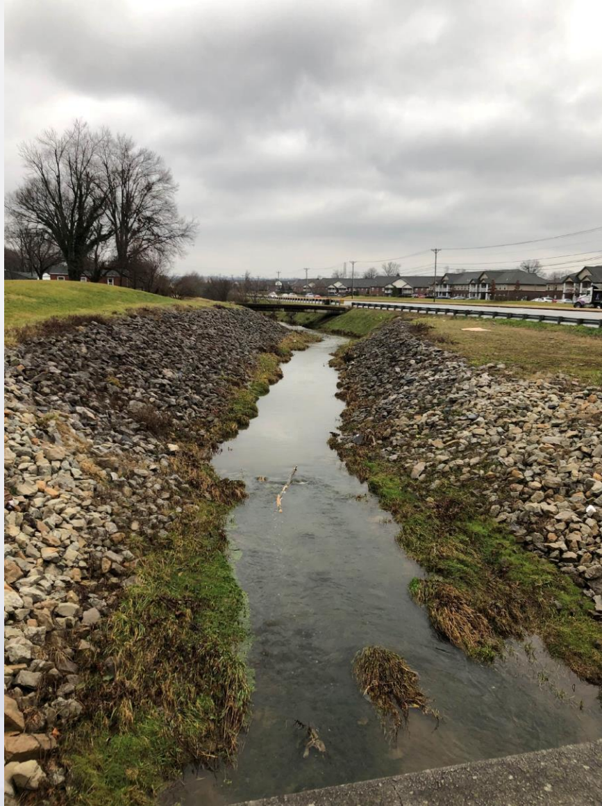
Location of Spring Ditch facing east.
