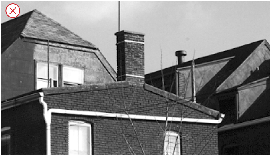
Install a gutter or downspout that is simple in design and that does not damage historic detail of the original structure.
