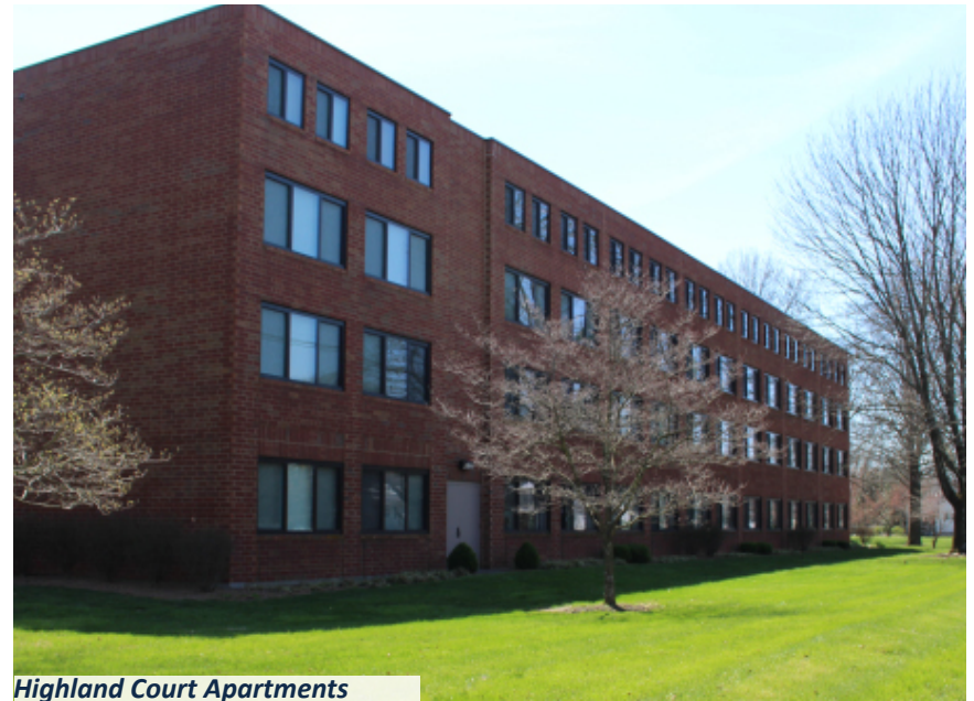
Highland Court Apartments
