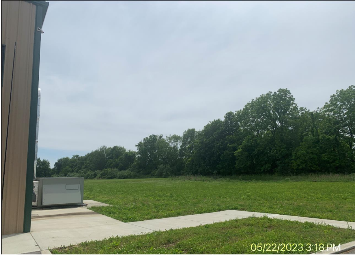
Area where second Multipurpose building will be built
