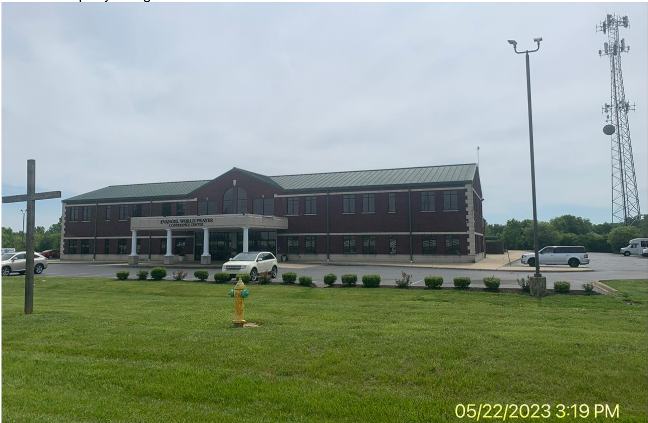
Front of Property along Billtown Road
