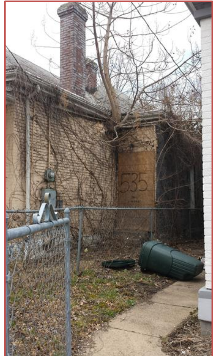
Exterior – East Side
