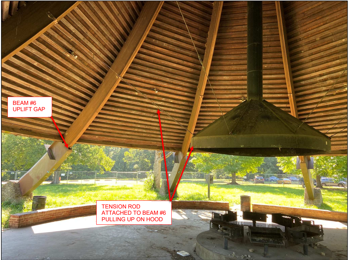
Photo 5: Hood Lifting from Beam #6 Movement
