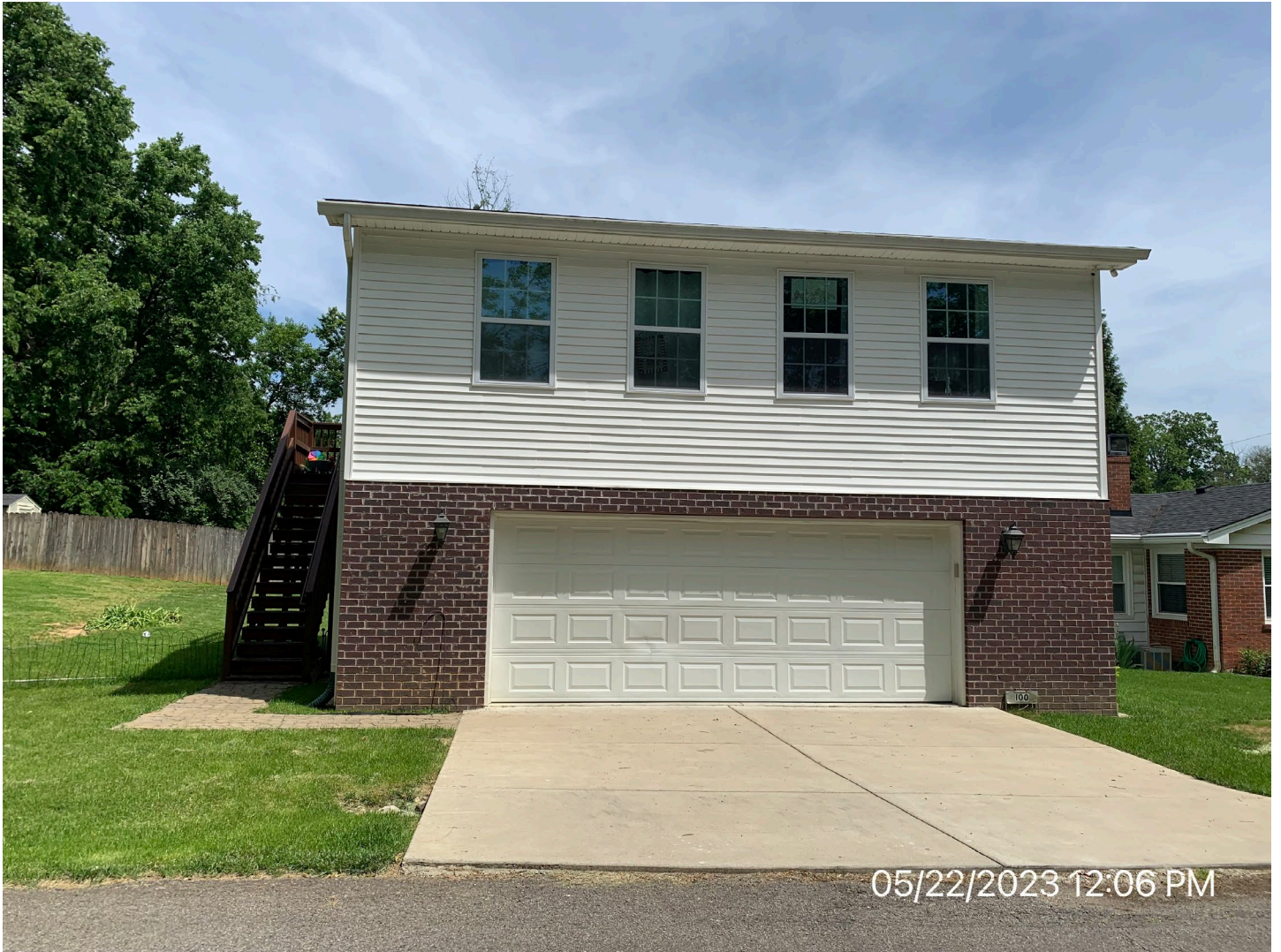
View of accessory structure from side street.
