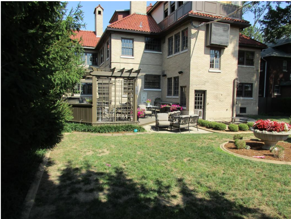
Looking toward rear of the Condominiums from the rear property line
