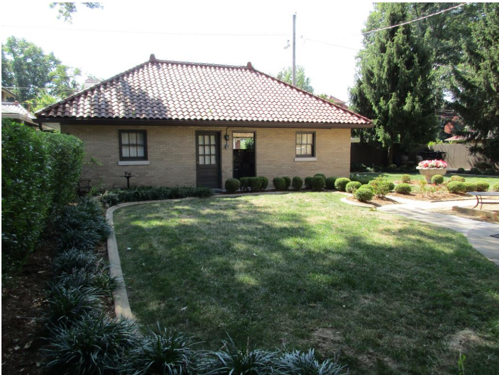
Existing east rear yard
