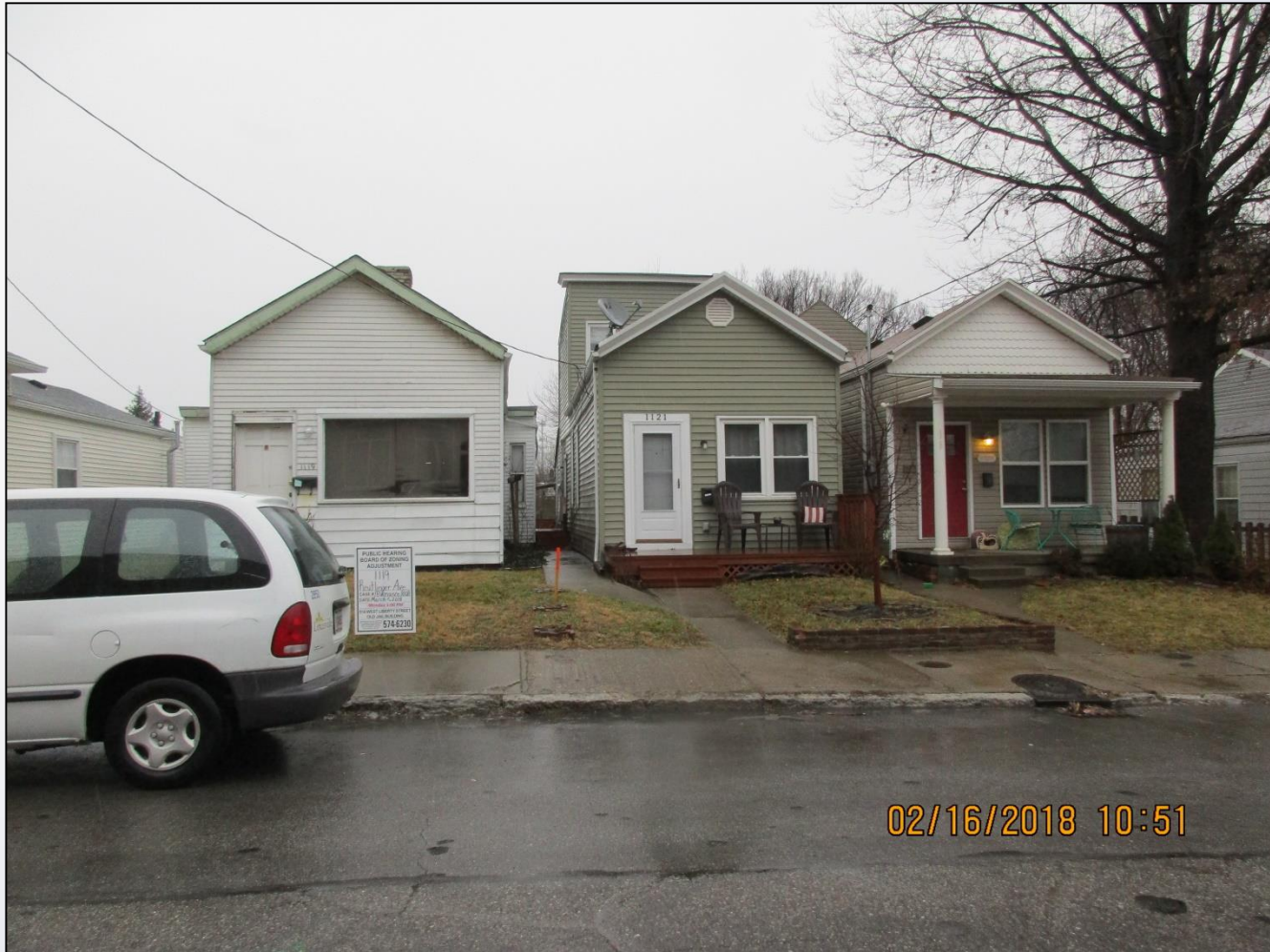
The front of the subject property and the property to the right.
