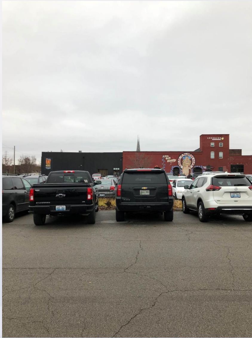
Western façade of subject property.
