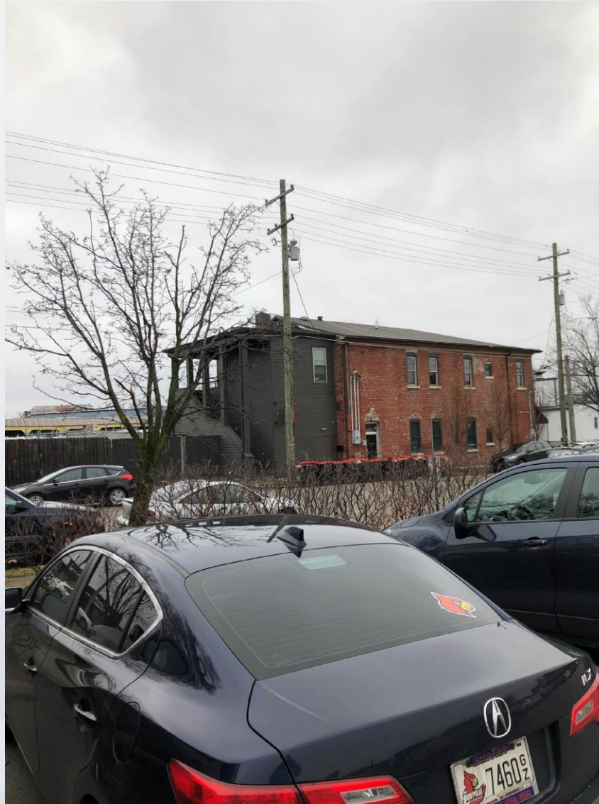
Property to the west.
