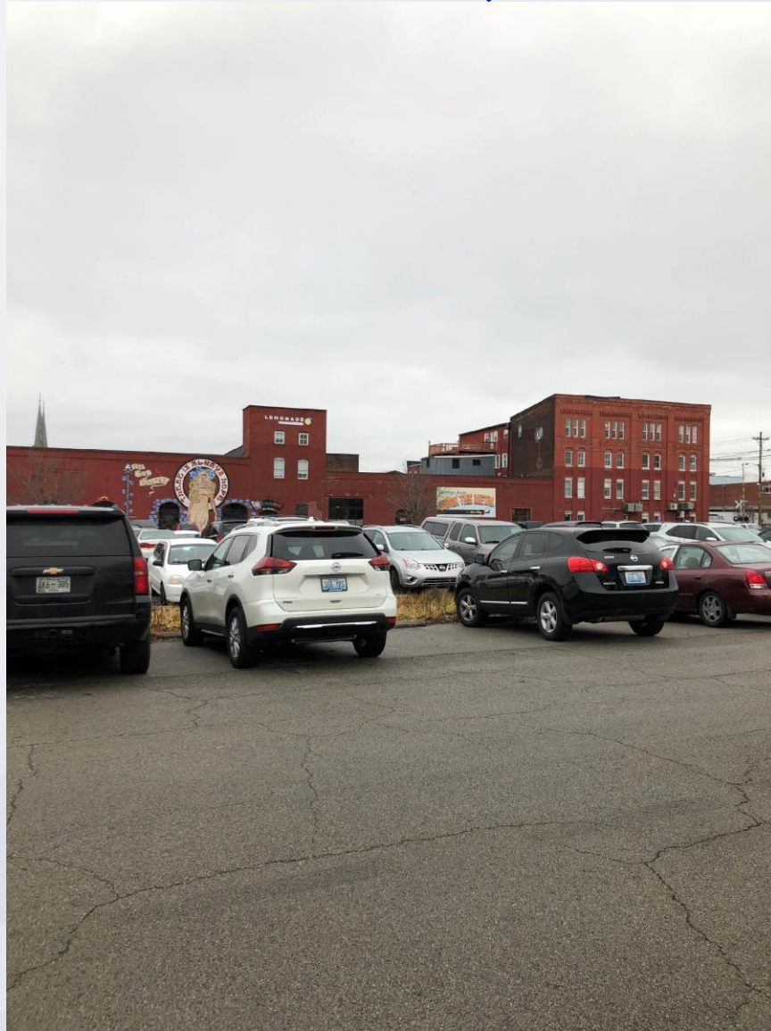
Western façade of subject property.
