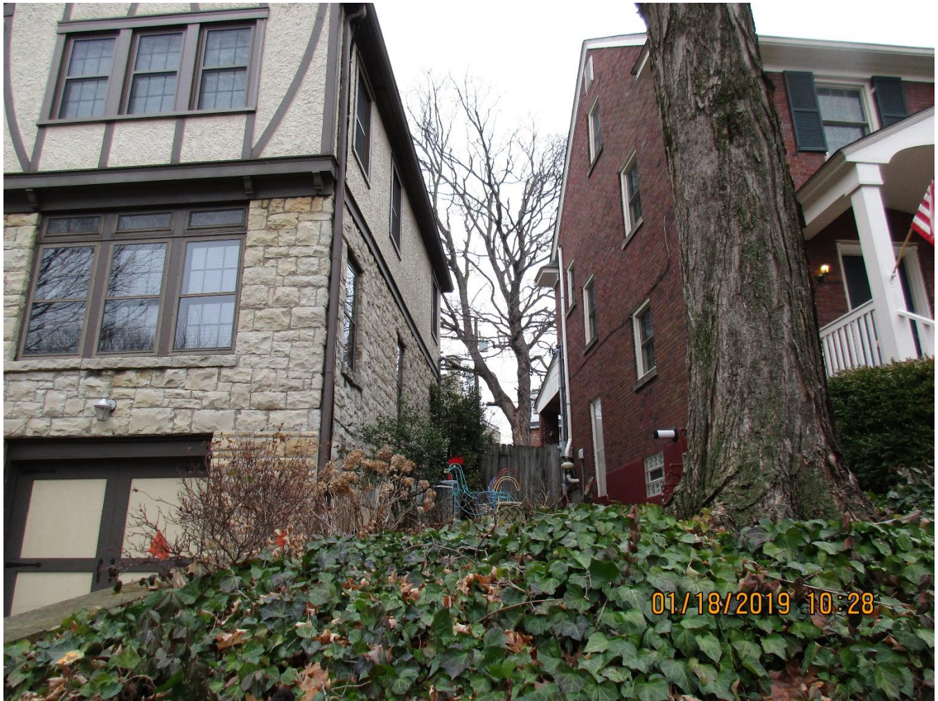
Side yard that is being encroached upon and property to the right.
