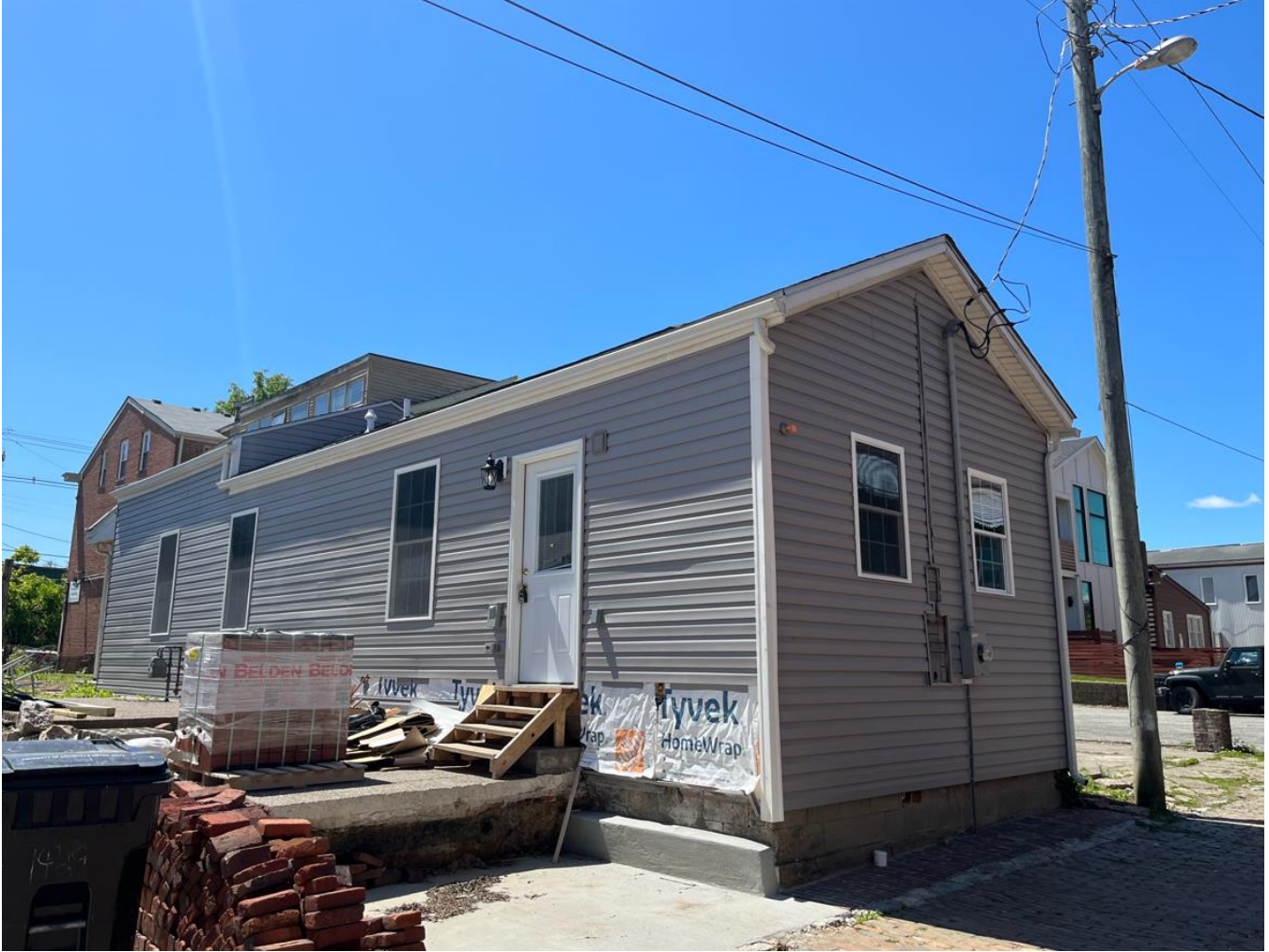
View of variance area for covered portico.
