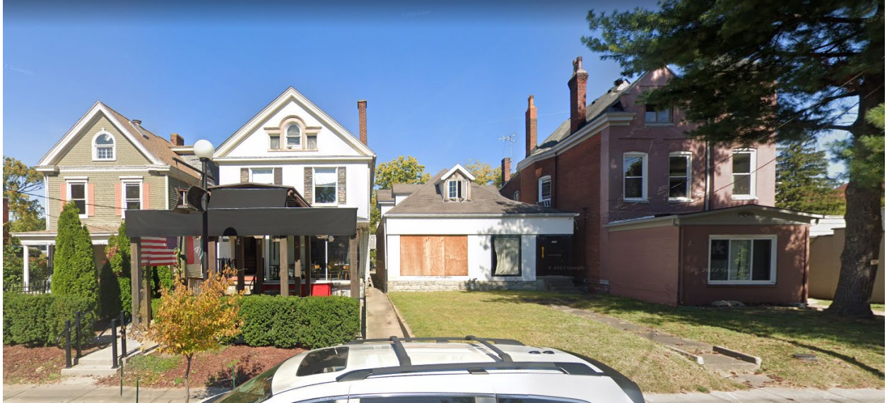
1331 Bardstown Rd. Adjacent Context - Google October 2022
