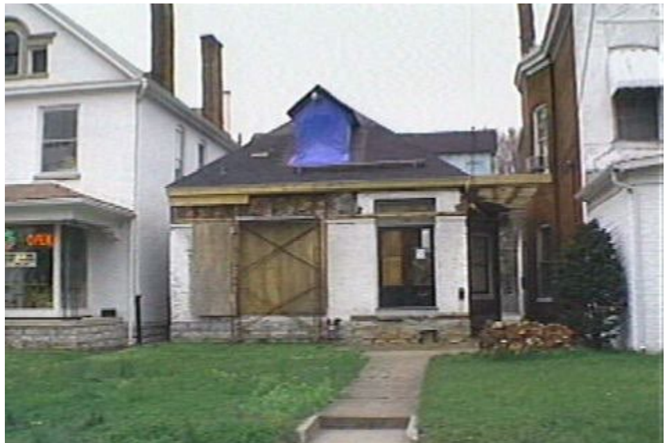
1331 Bardstown Rd., Past Context – PVA 1999
