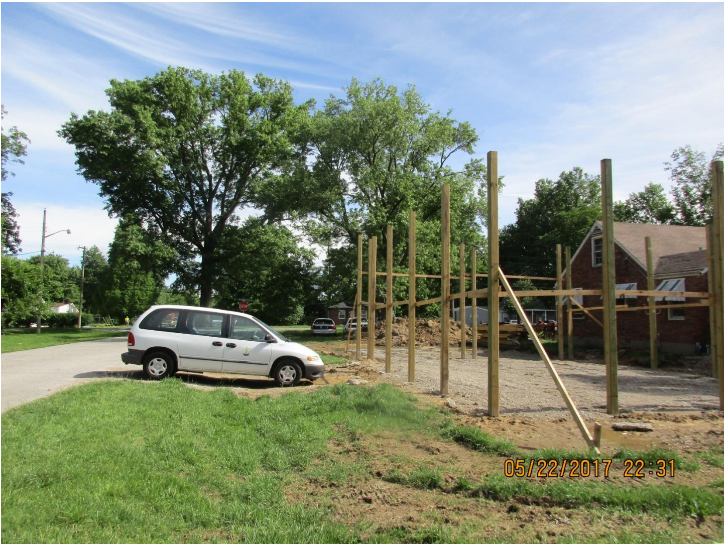
Looking north along the western side of the pole barn.
