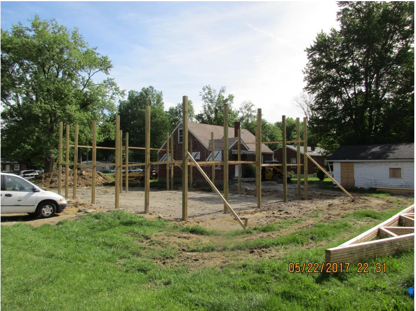
The south-west corner of the partially constructed pole barn.
