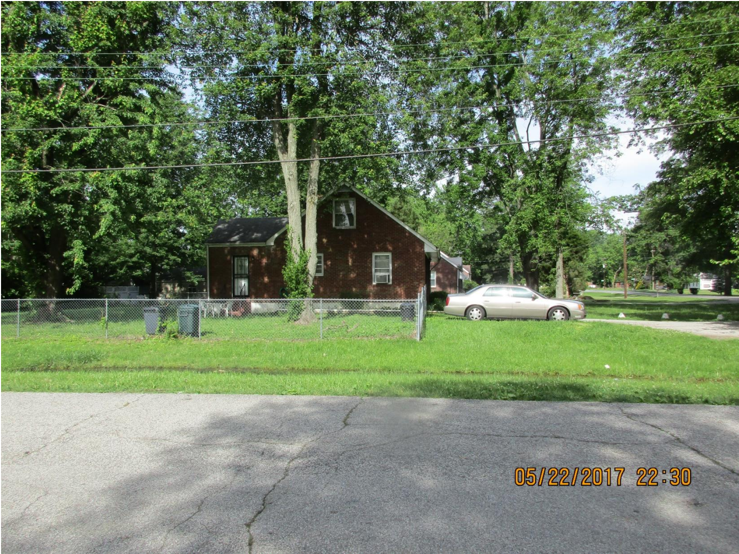
The residence across Daleray Drive.
