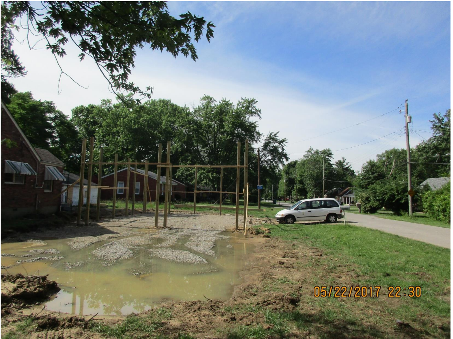
Looking south at the front of the pole barn.
