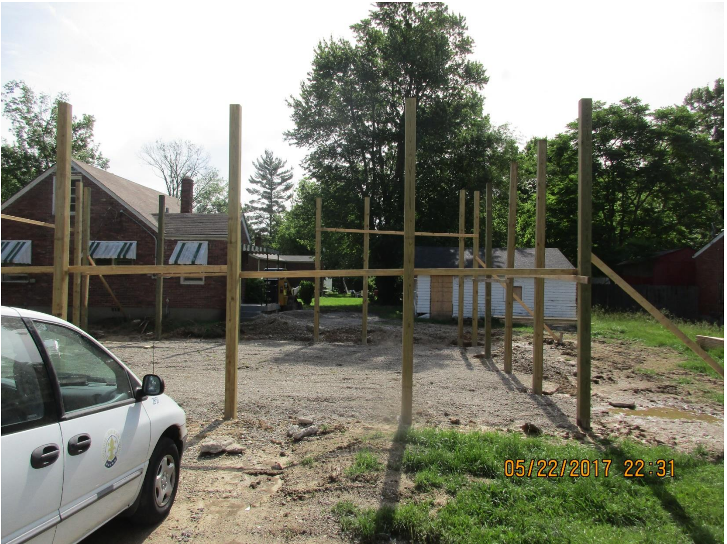
The partially constructed pole barn.
