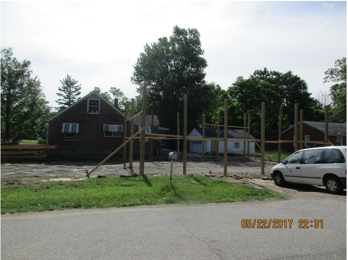
The partially constructed pole barn as seen from across Daleray Drive.
