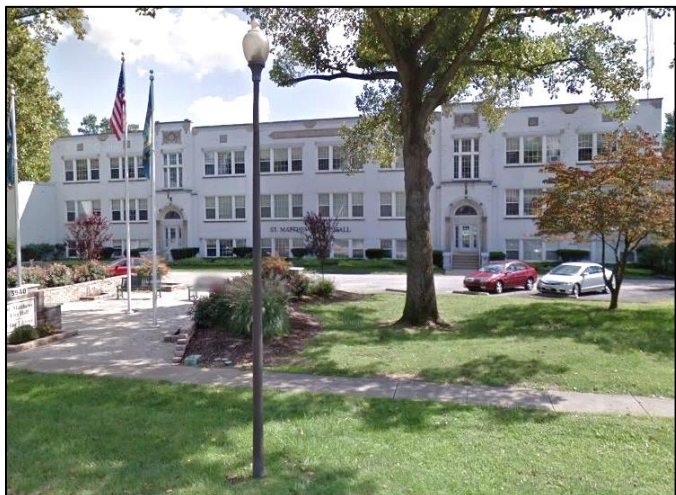
Figure 54. Greathouse School, 3940 Grandview Avenue (Google)
