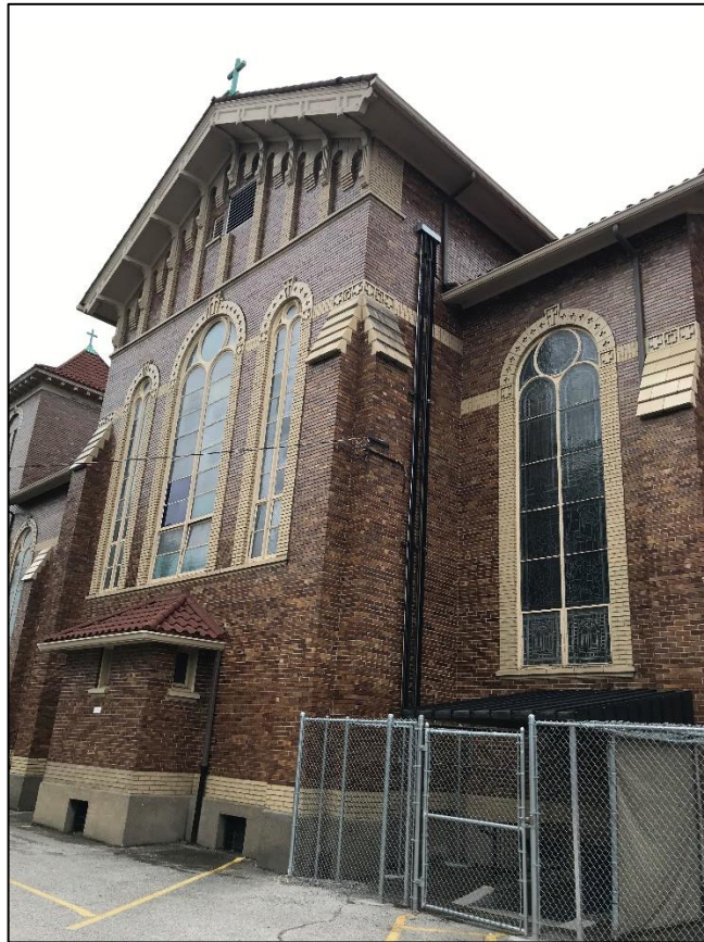
Figure 5. North elevation of Building 1, looking southeast.
