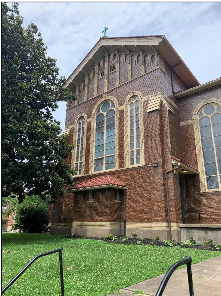
Figure 6. South elevation of Building 1, looking northwest.
