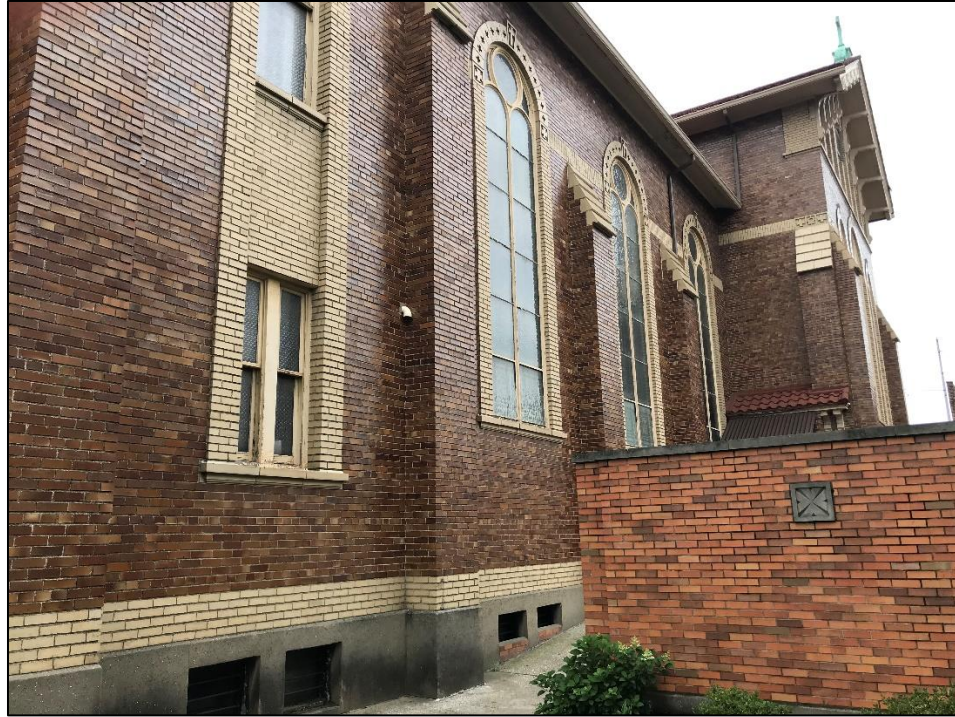
Figure 4. North elevation of Building 1, looking southwest.
