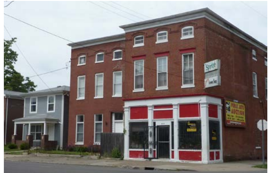
Typical corner store building with housing above and next door
