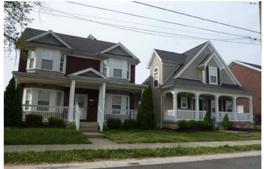
Recent housing construction in Russell
