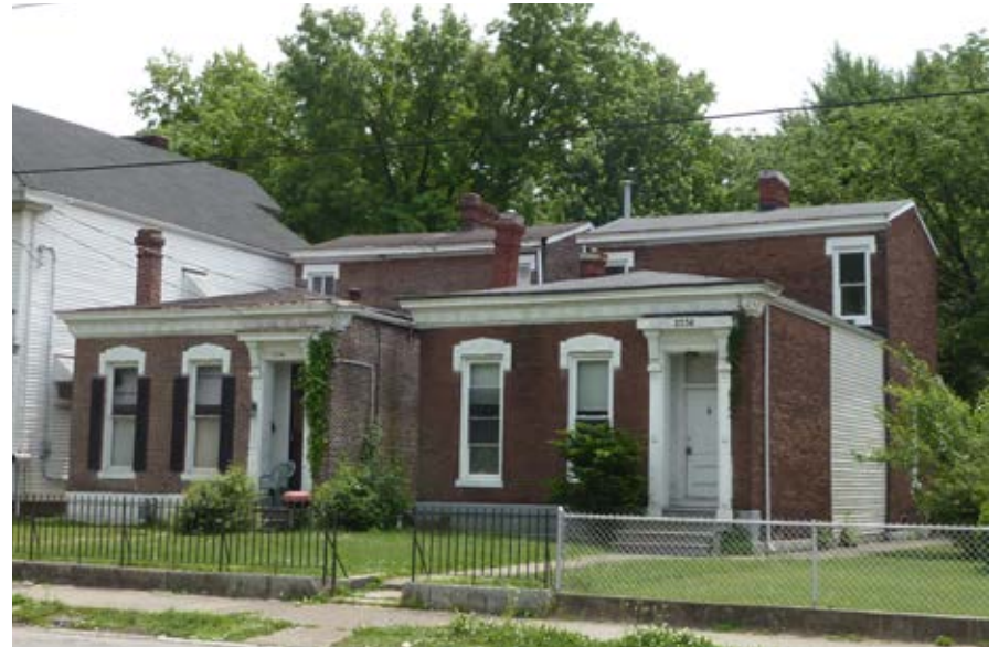
Shotgun houses with common "camelback" rear additions
