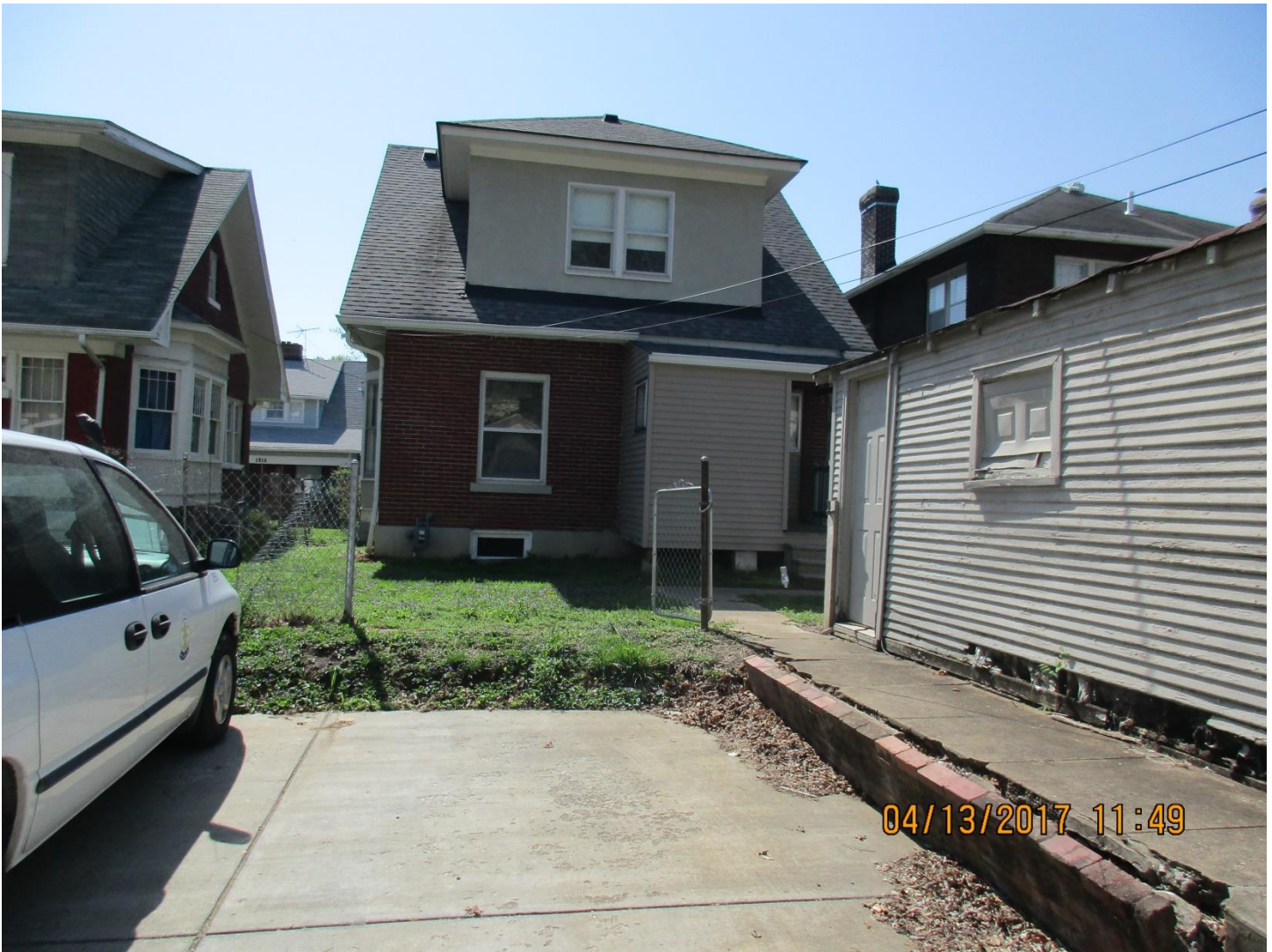
The rear of the property, where the addition is to be built onto the house and where the garage is to be constructed.
