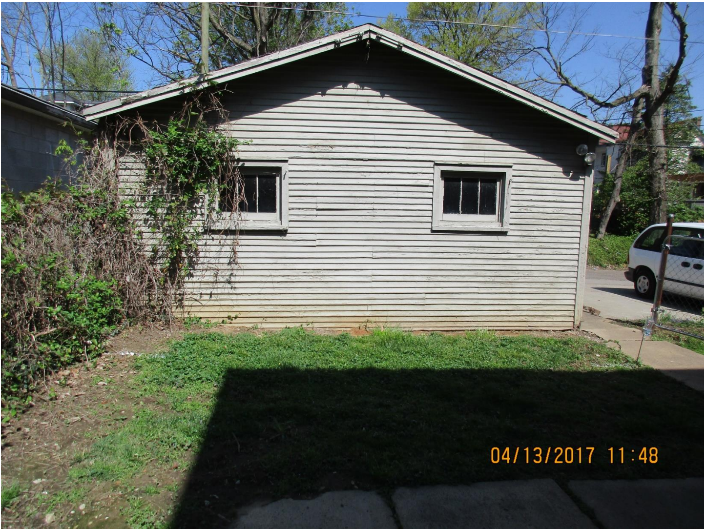
The existing garage to be removed.
