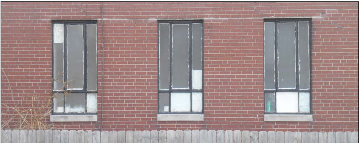
Rear facade windows
