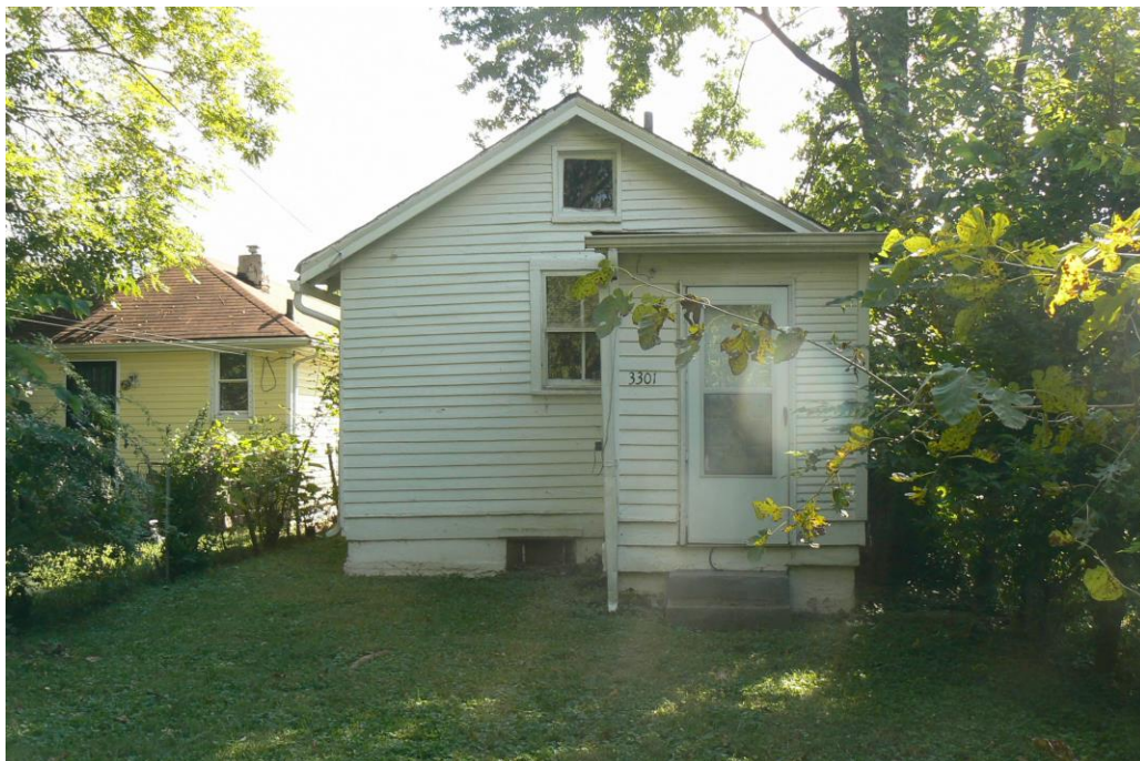
Rear view – 3301 Greenwood Avenue
