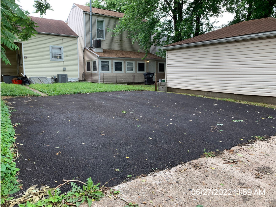
Parking pad at rear of property
