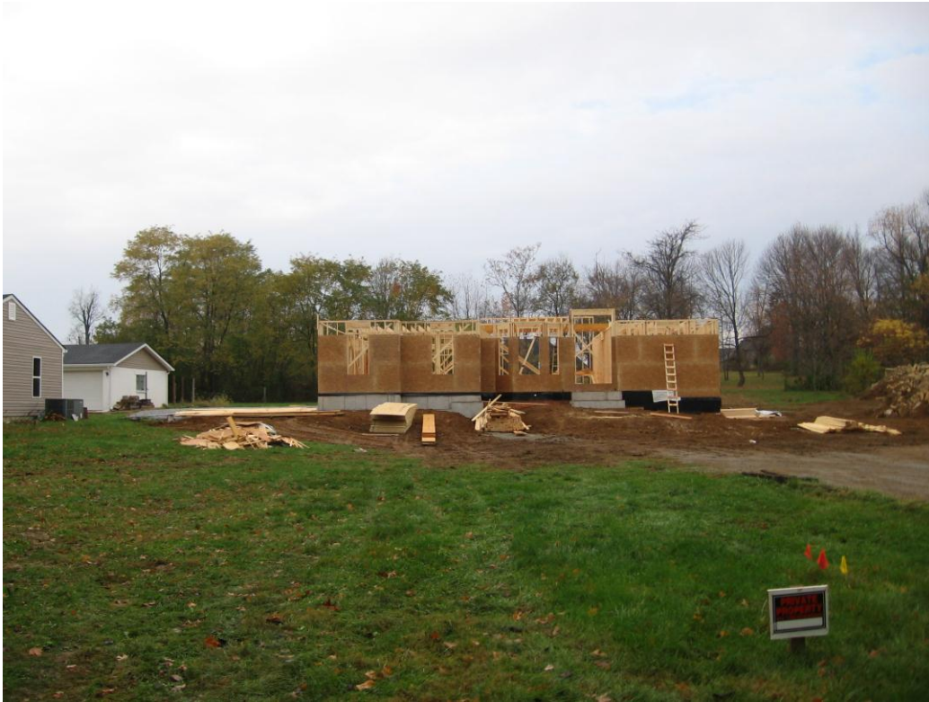
New house under construction
