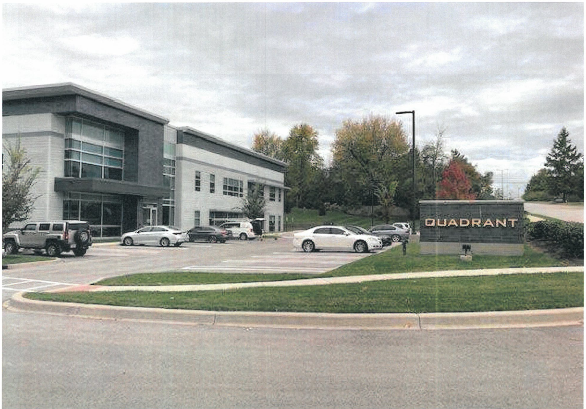
View of existing Quadrant facility.
