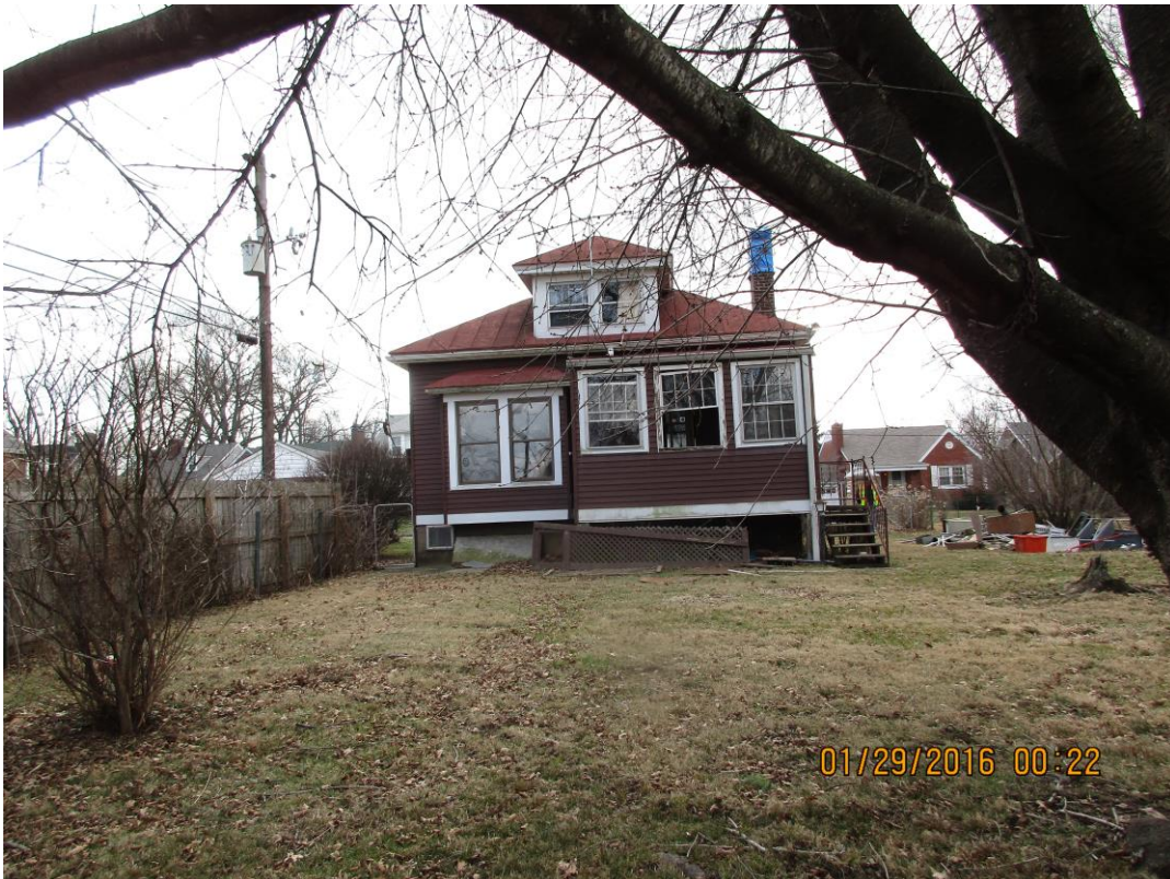
Looking at the rear of the principal structure where the new rear addition would be built. (Looking SE)
