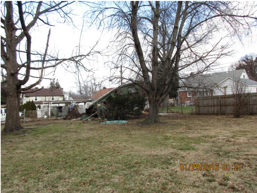
Rear Yard where the existing dilapidated garage has fell and where the proposed garage would be placed (looking N)
