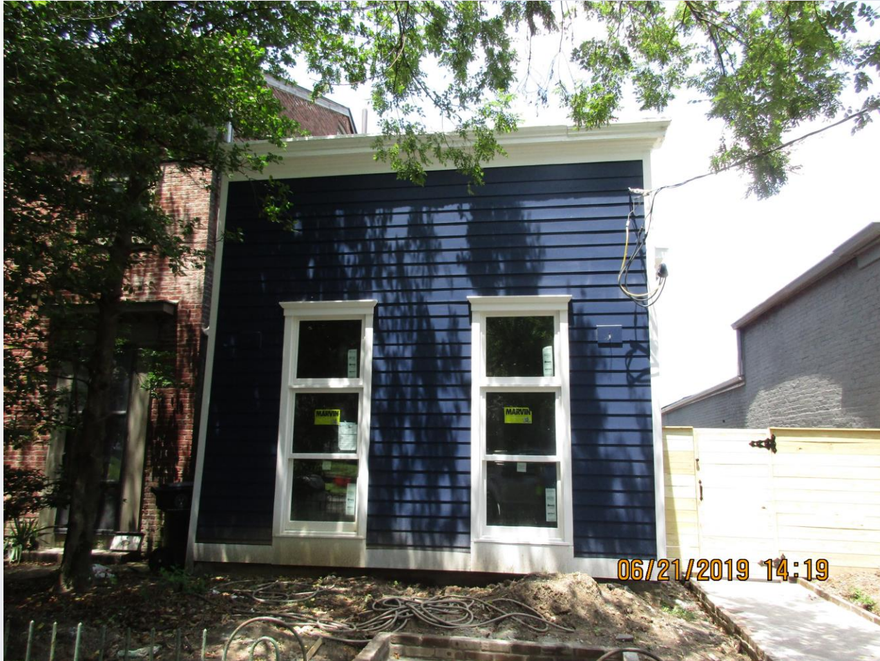
Front of subject property.
