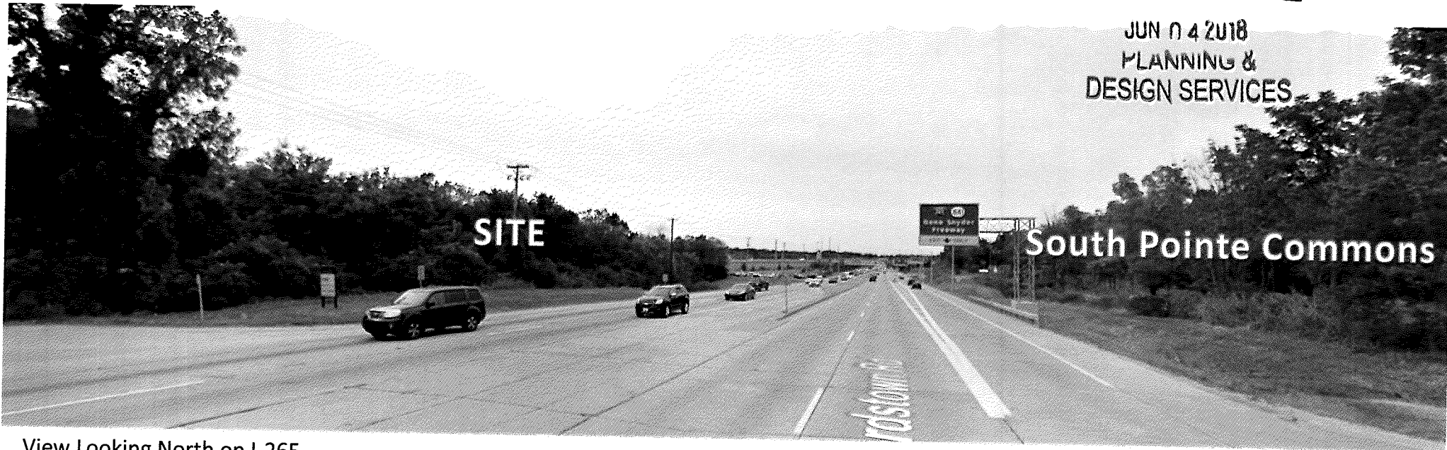
View Looking North on I-265
