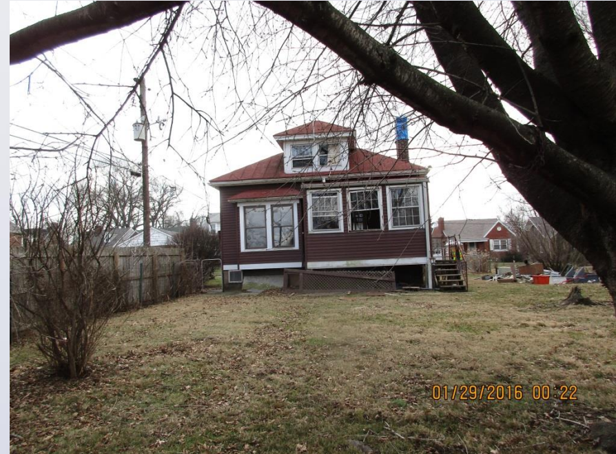
Looking at the rear of the principal structure where the new rear addition would be built. (Looking SE)
