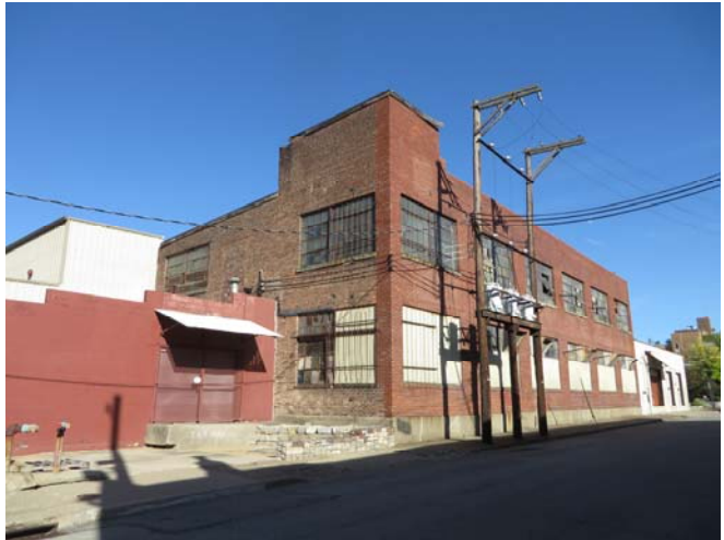
West façade, along Brent Street
