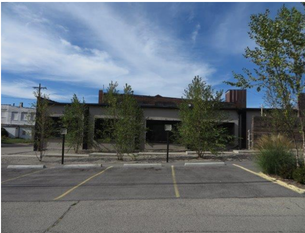
South façade, Louisville Stoneware Parking
