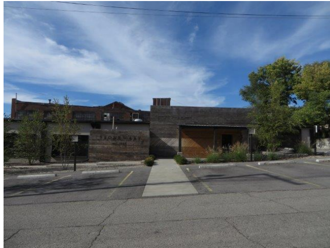
South façade, Louisville Stoneware entrance
