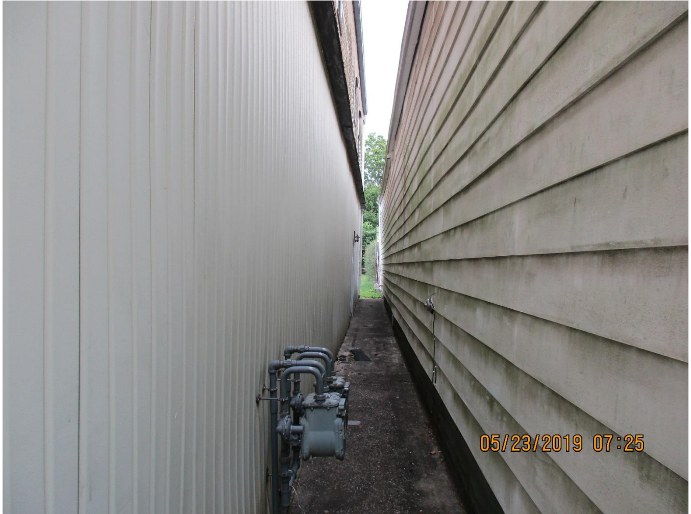
The western side of the subject property.
