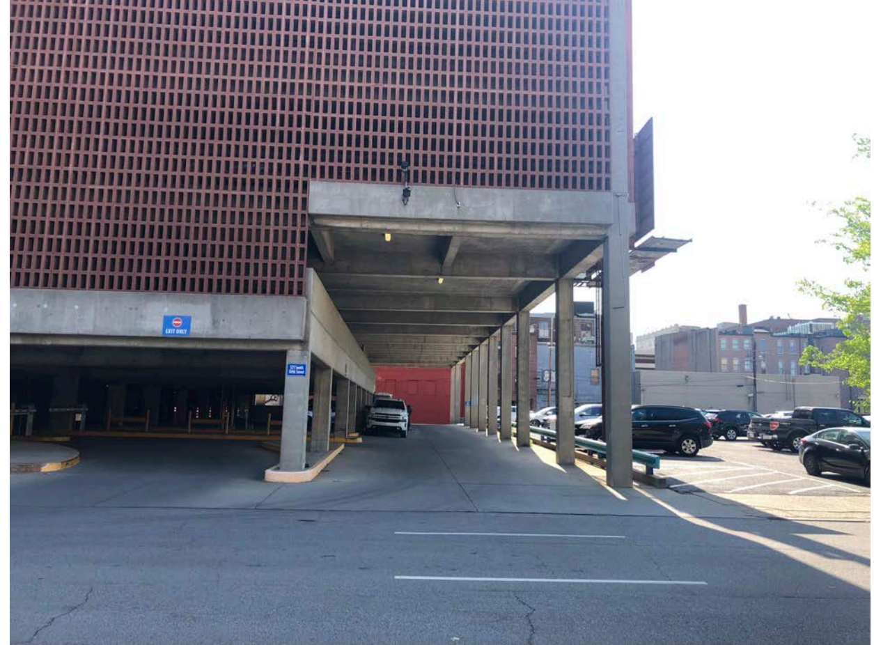
Service drive at Seelbach Garage
