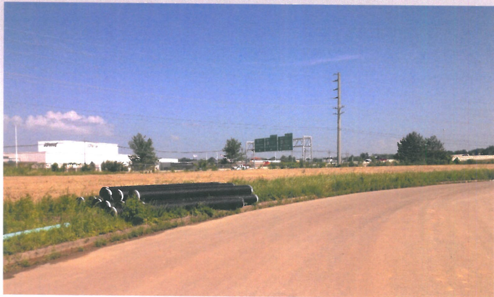
View of Watterson Expressway
