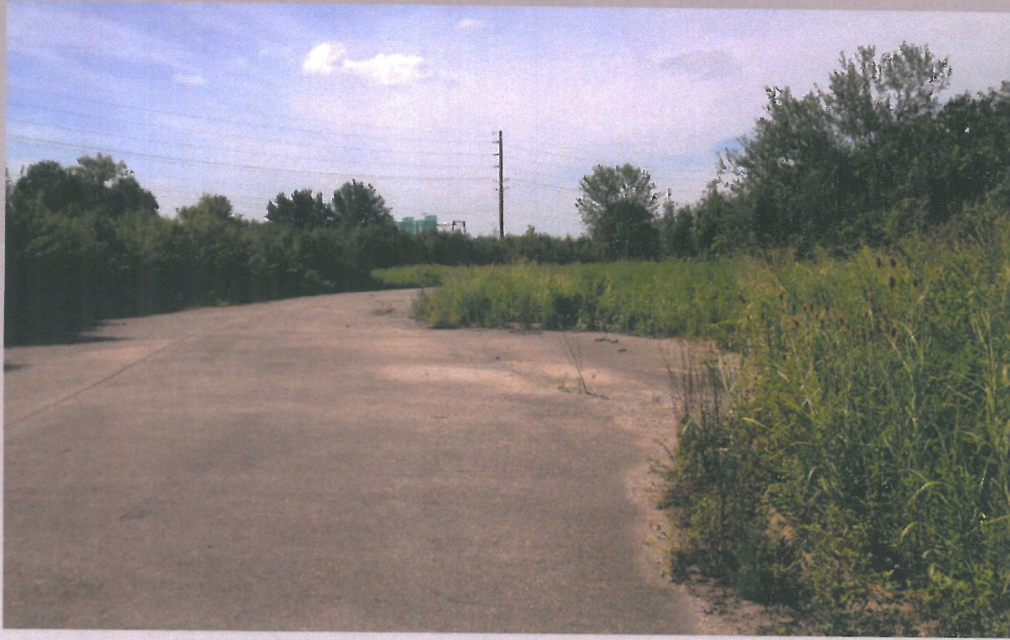
View of Existing Bullitt Lane
