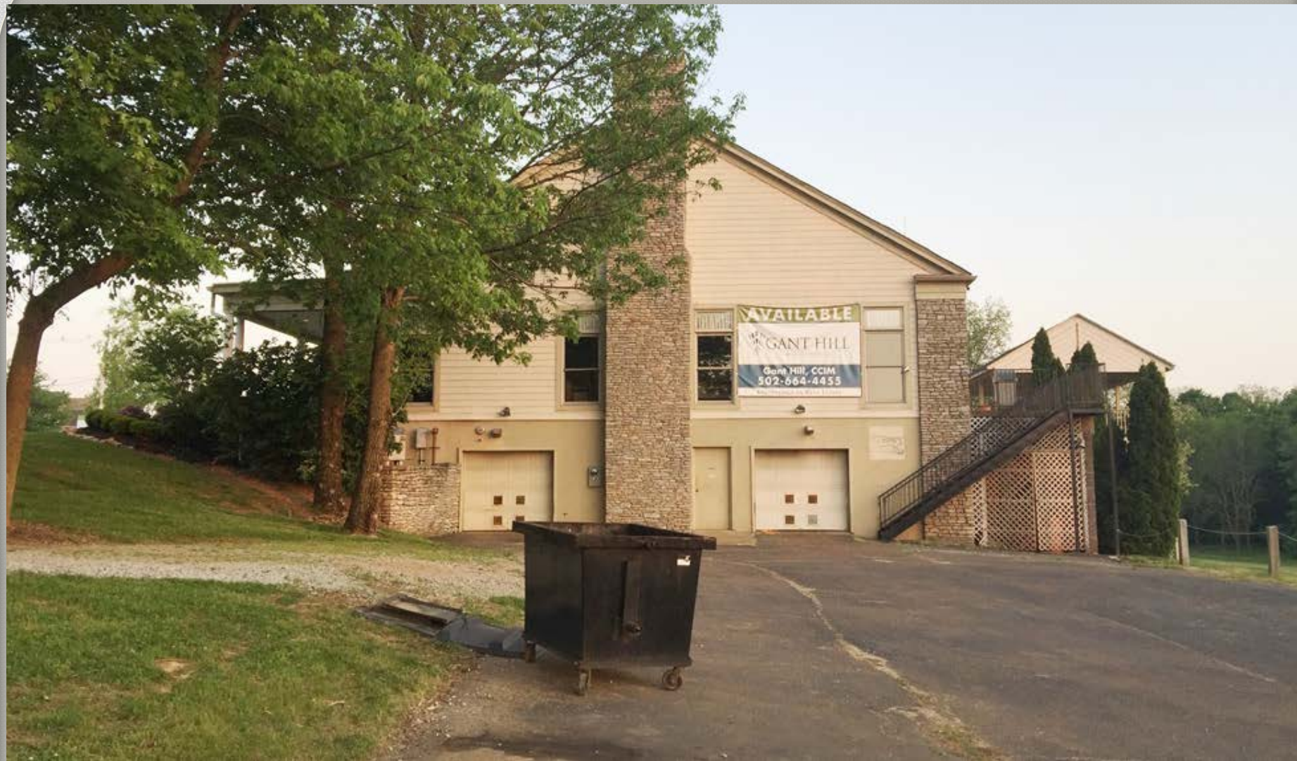
View from Westport Road side of the existing clubhouse.
