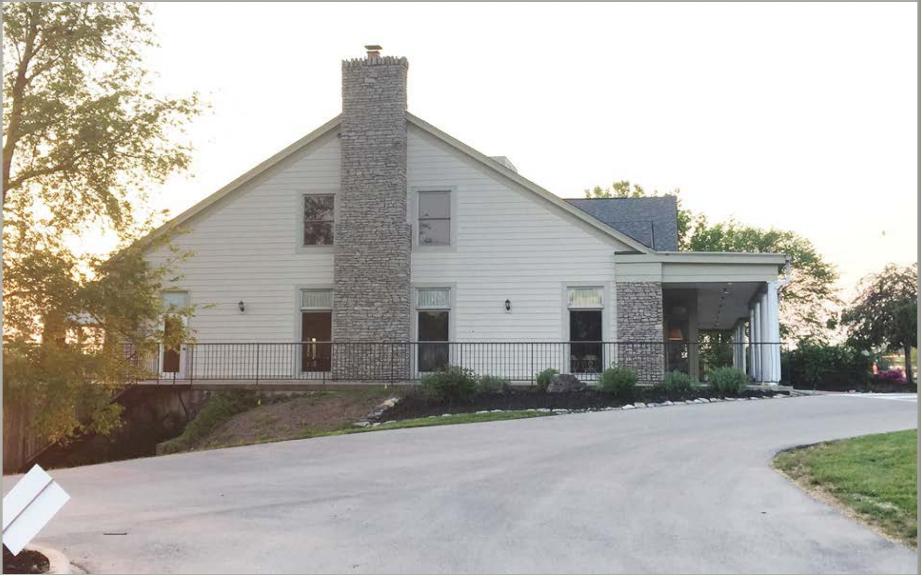
View from parking lot side of the existing clubhouse. Exterior of the building will remain mostly the same.
