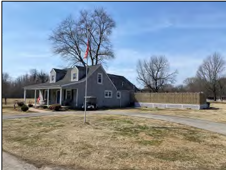
Photo 16. Front of house on subject property Photo facing southwest
