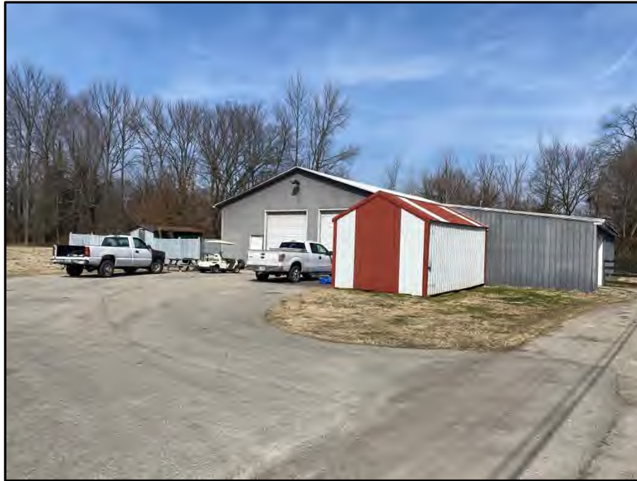
Photo 17. Front of garage on subject property Photo facing north
