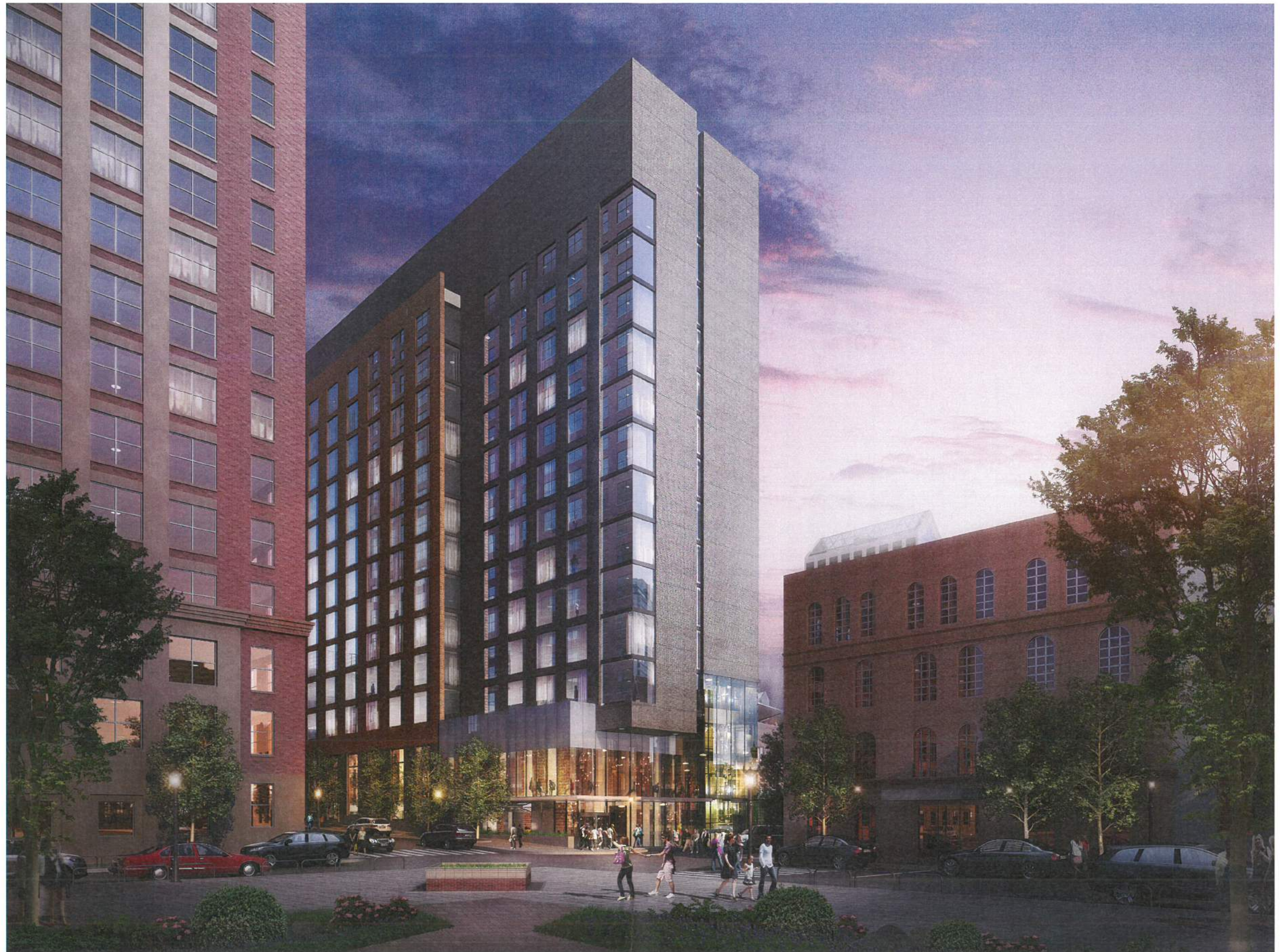
VIEW AT MAIN ST & N. FIRST ST
