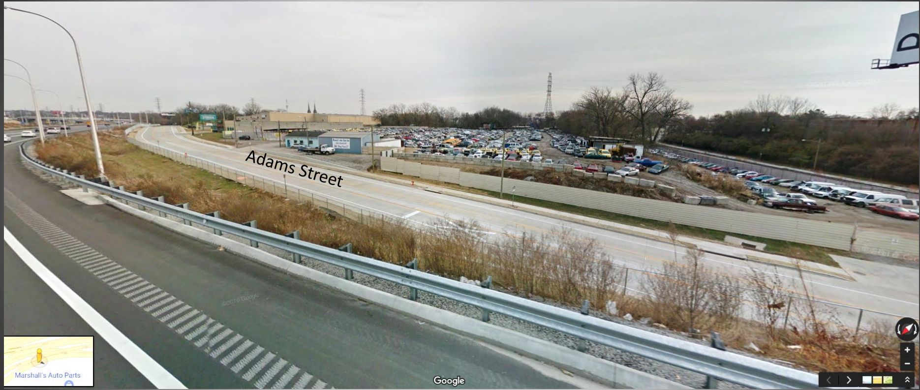
View of site from I-71, looking southeast.
