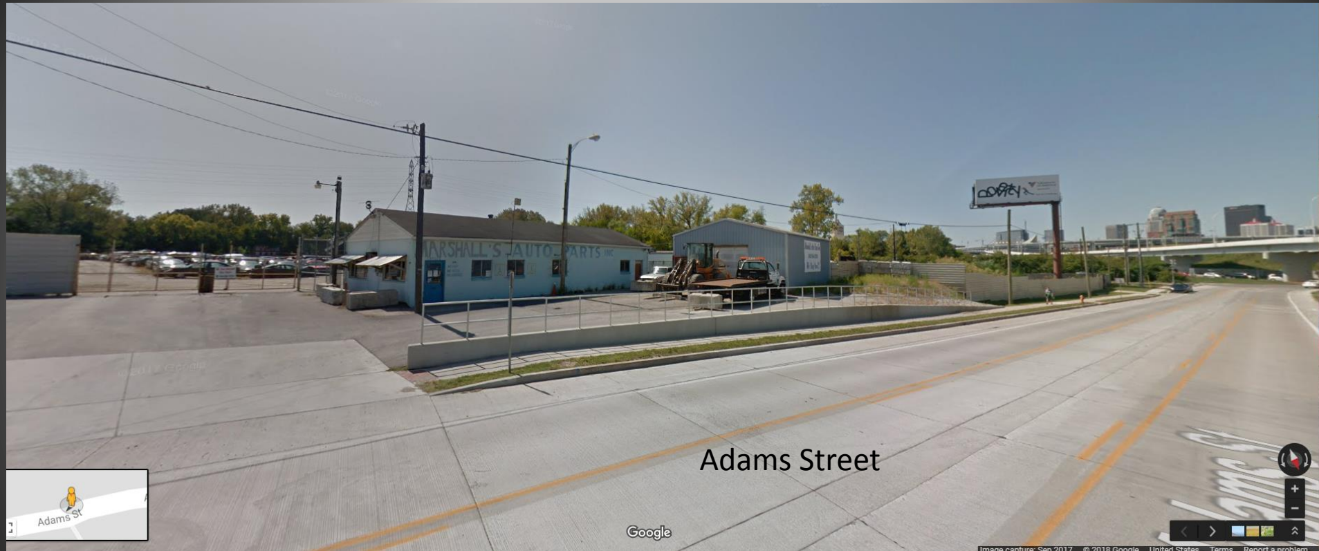
View of existing Marshall's Auto Parts from Adams Street, looking southwest.
