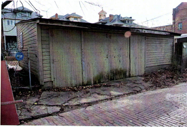
Current garage structure:
