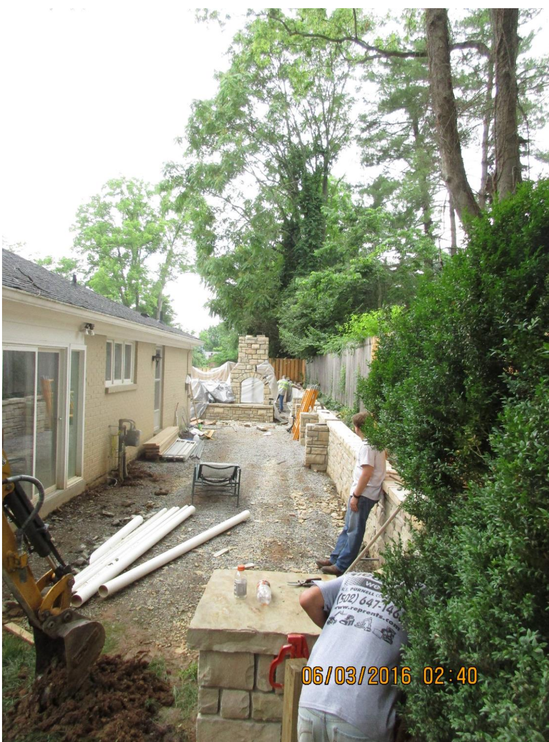
Looking at the front right hand side of the property where the proposed roofed outdoor living would be constructed the proposed length along this side of the house is approximately 35'. The pitched roof would be supported by the wall you see in the right of the photo.
