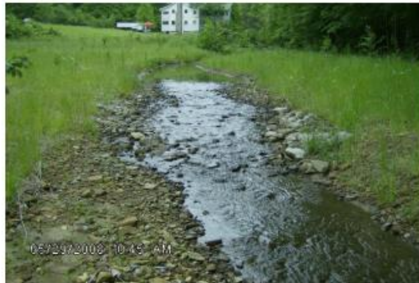
Below: Stable stream with high habitat value and no erosion after restoration.
