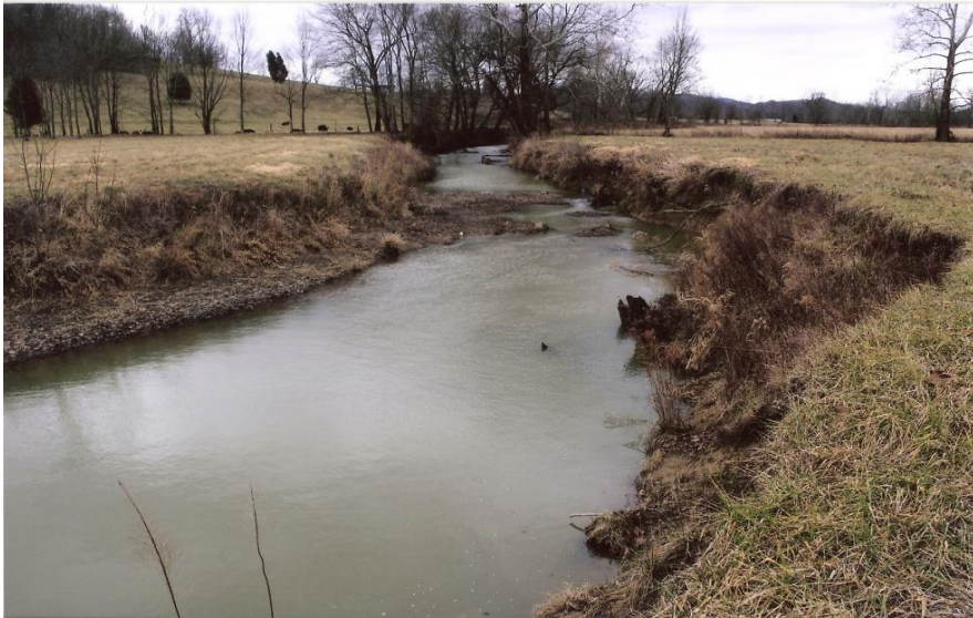
Eroding banks (above); stable stream banks and in-stream habitat restored by the FILO program (right)
