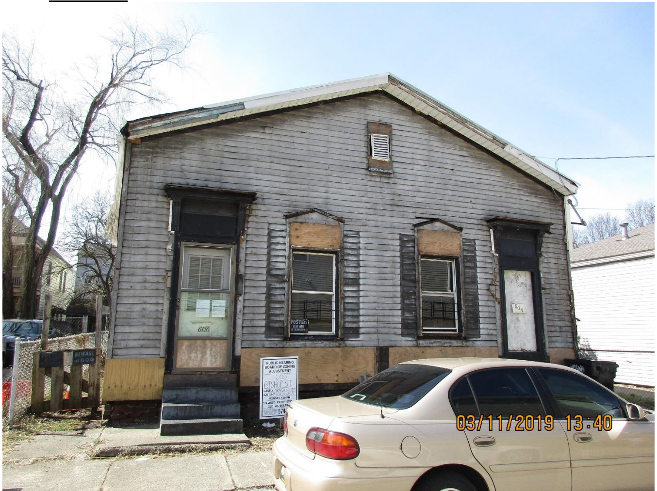
Front of subject property.
