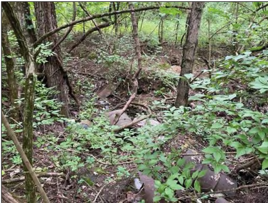
PHOTO NO. 2: Sinkhole – north central portion of site
