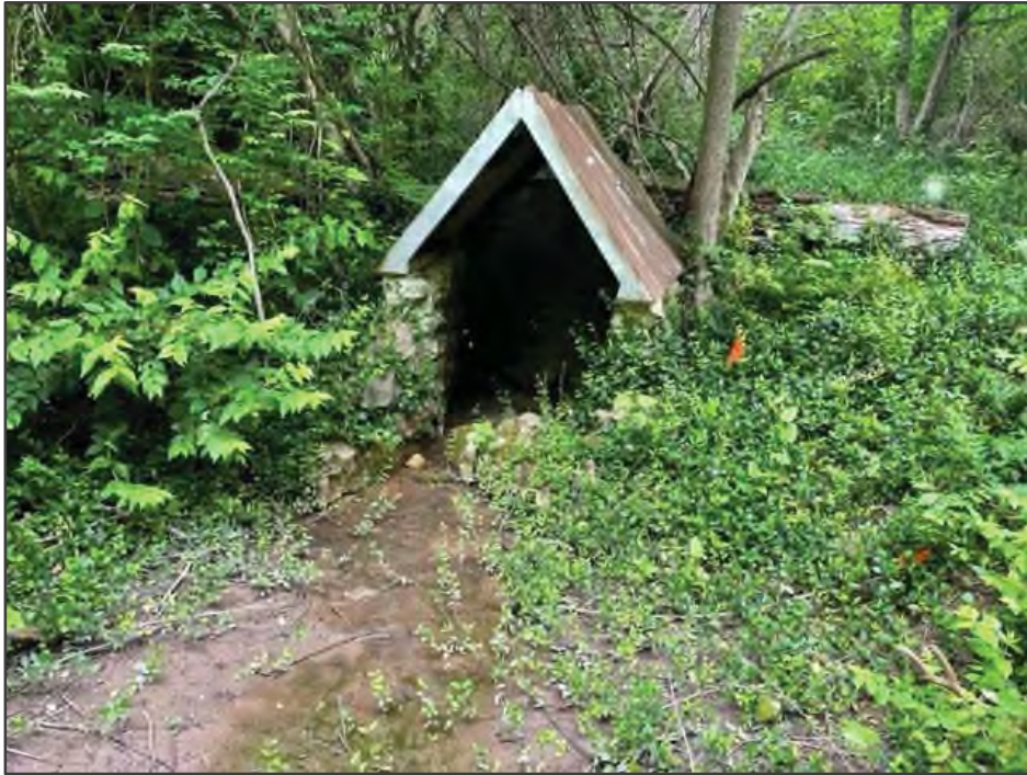
PHOTO NO. 5: Springhouse near southwest corner of useable area
