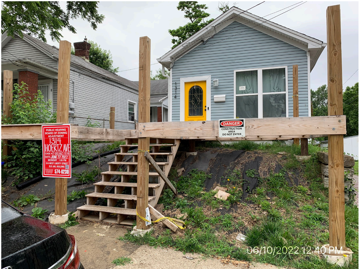
Front of subject property and variance area.
