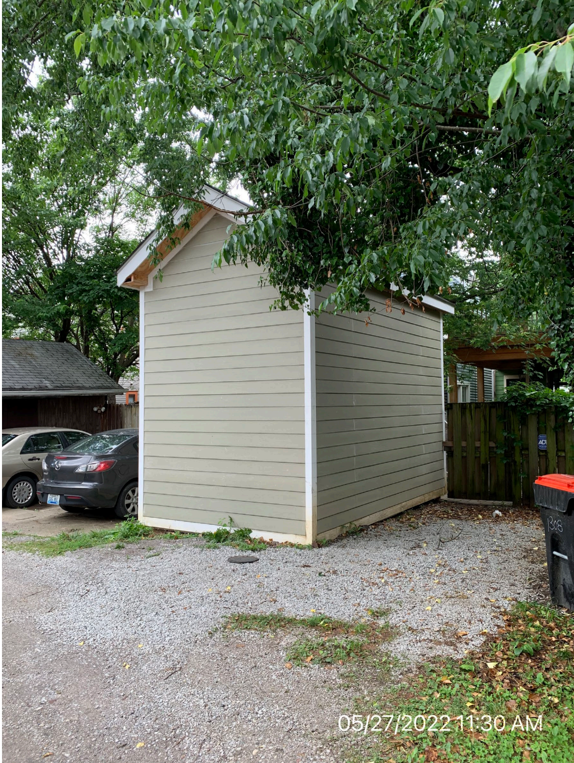
View of accessory structure from alley.
