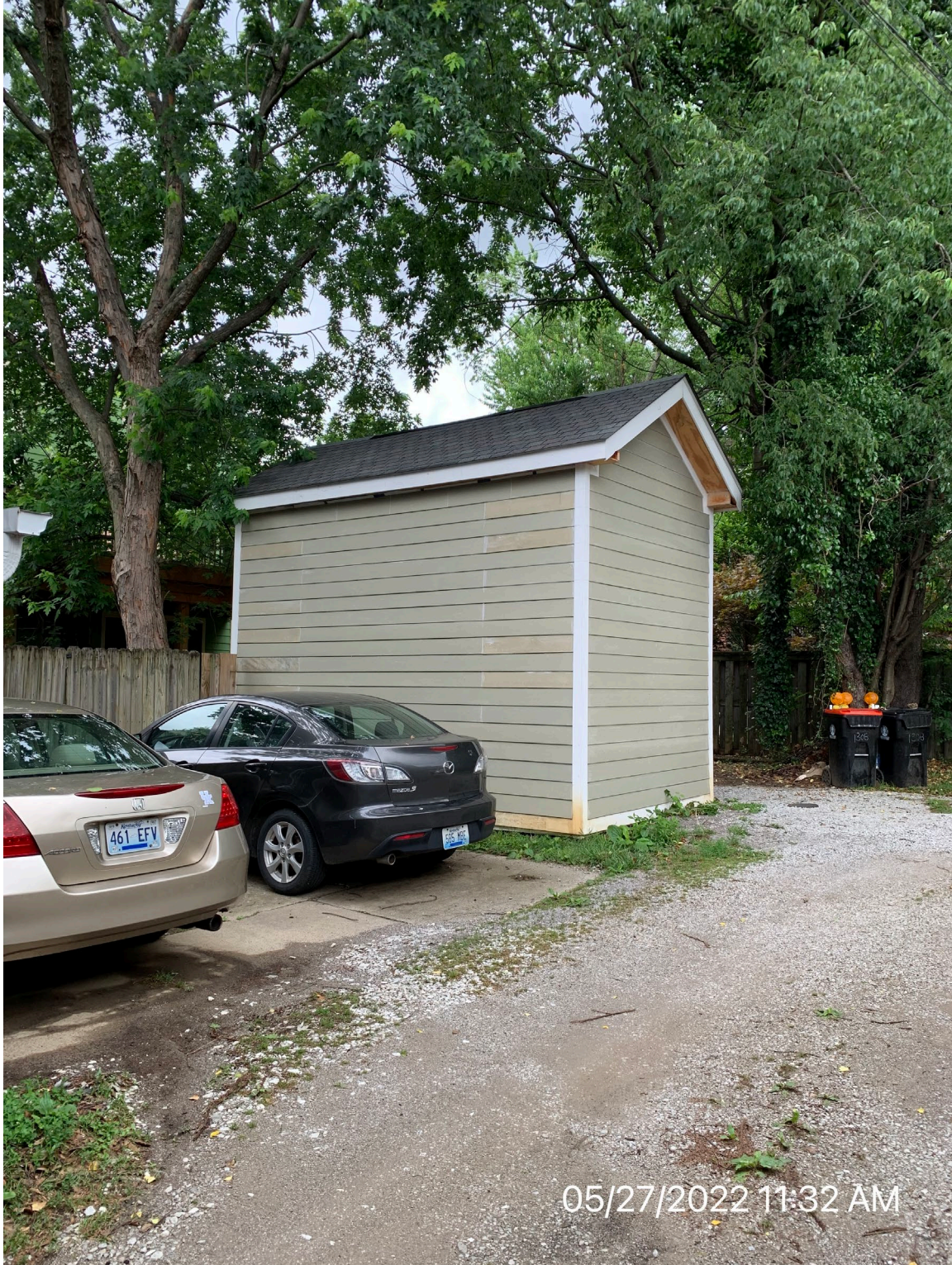
View of accessory structure from alley.
