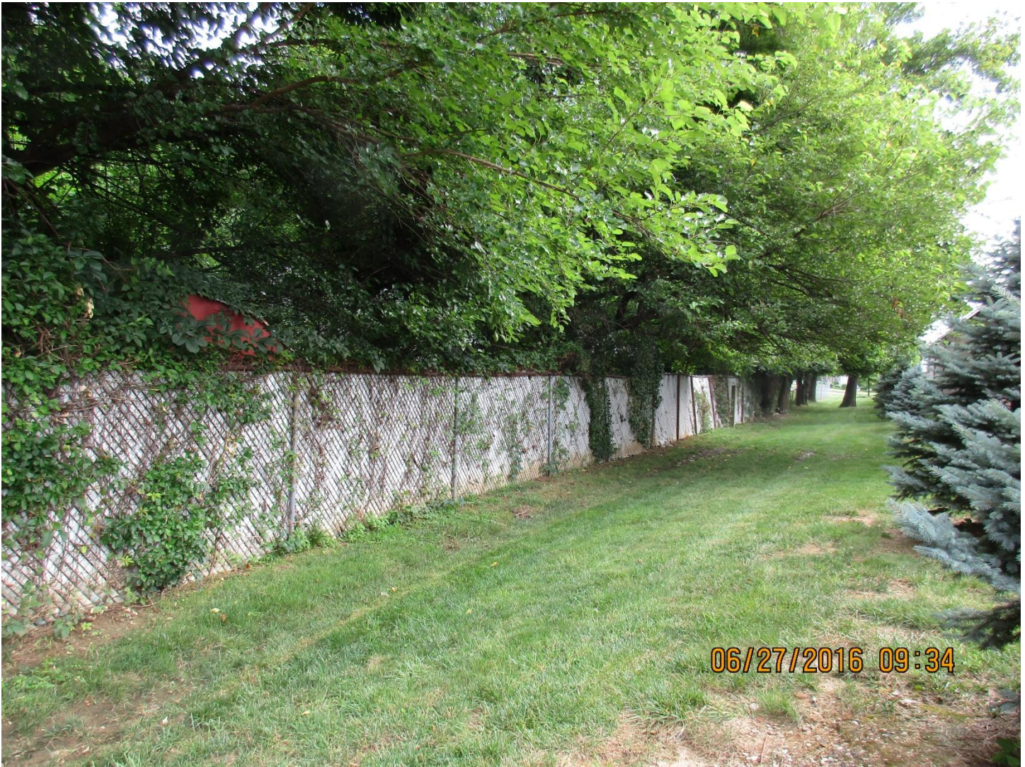
The eight foot chain link fence with screening strips and the trees for screening. A four foot unscreened chain link fence is located further North (center left of photo) at the rear of residential properties.
