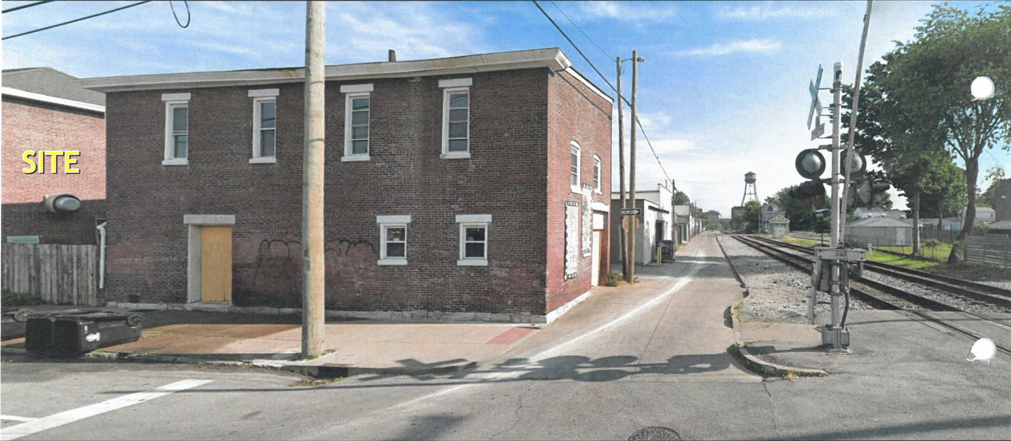
View of alley behind site
