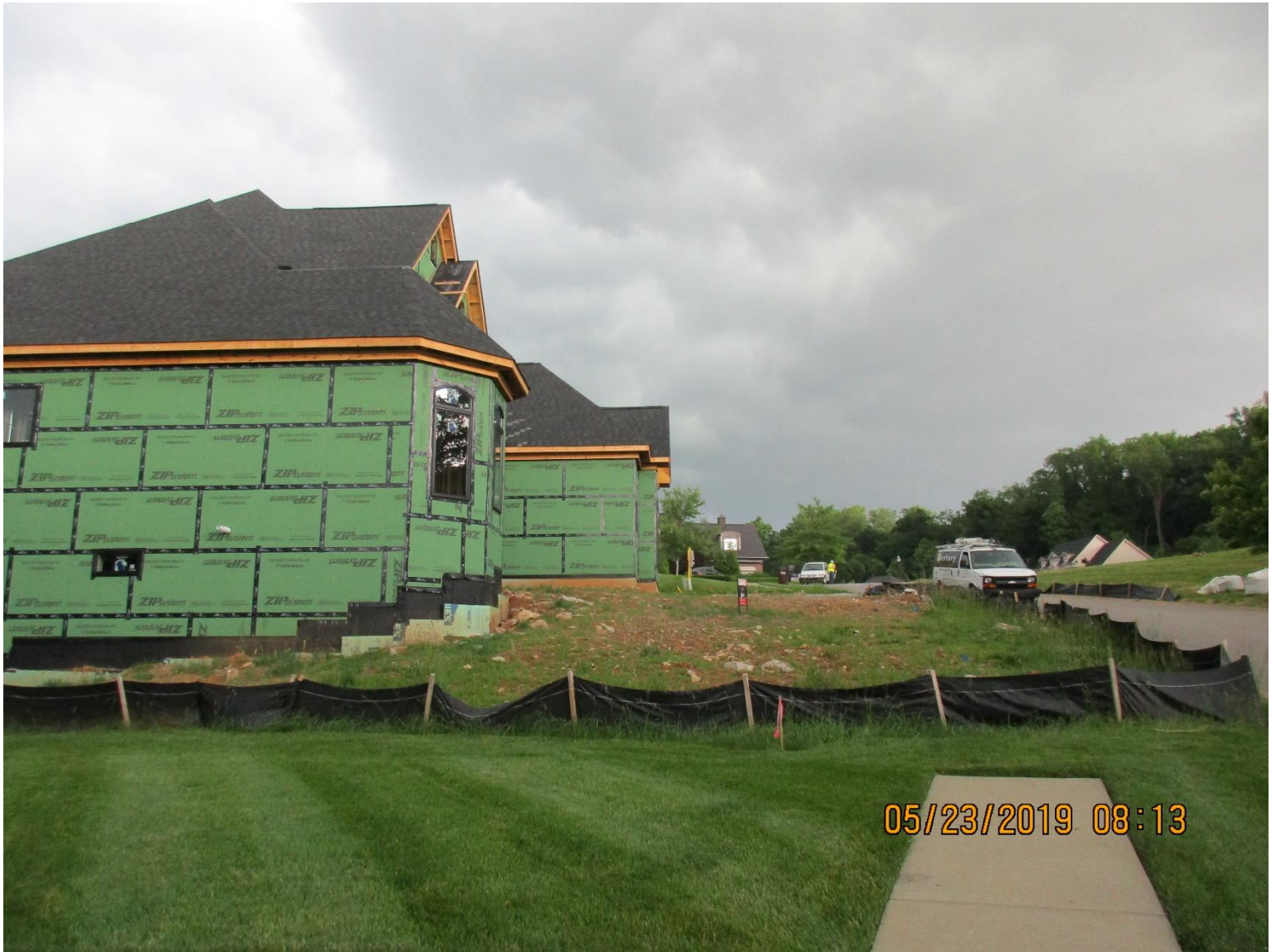
Looking east showing the front yard setback.
