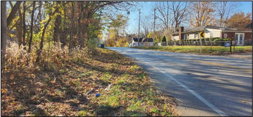
VIEW TOWARDS SOUTH N ENGLISH STATION RD
