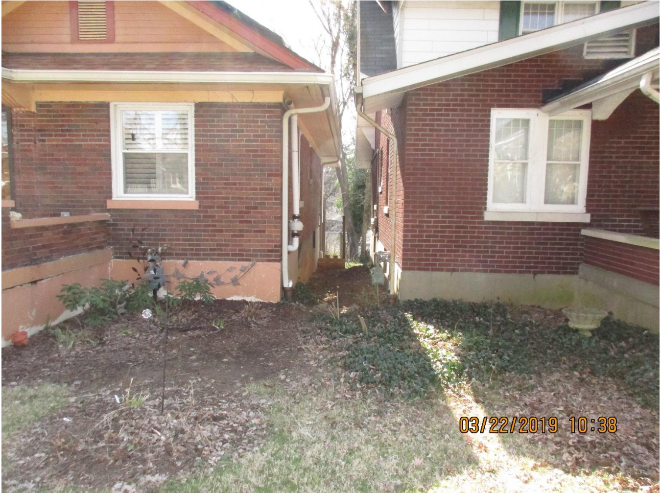
Side property line that is being encroached upon.
