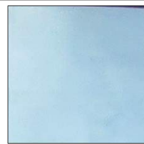
GLAZING - EXISTING CURTAIN WALL
