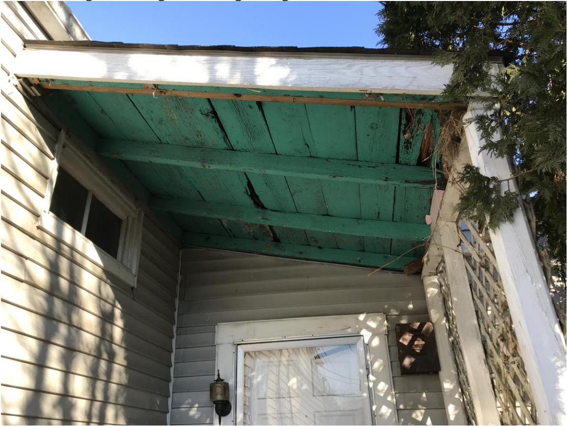
Side door porch roof framing.
