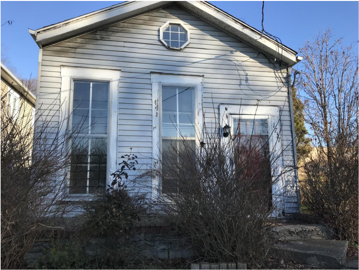
Front Elevation of Building
