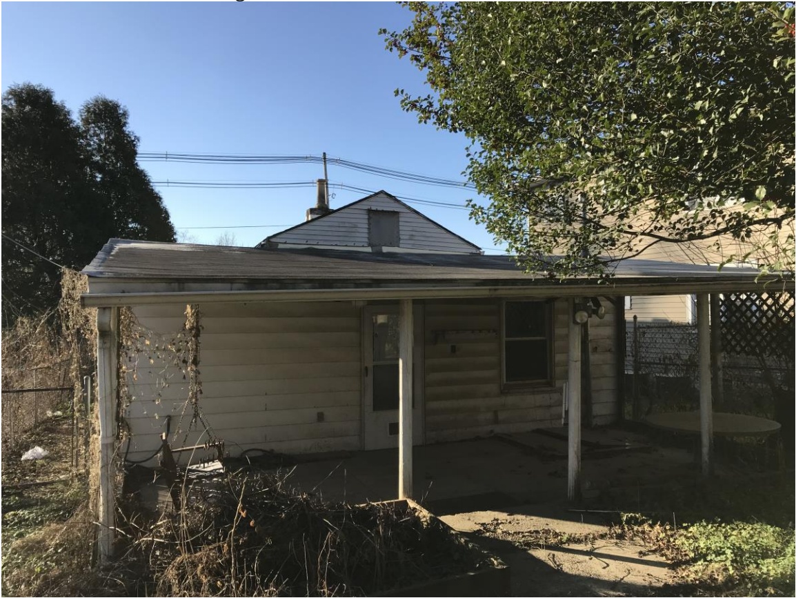
Rear Elevation of Building
